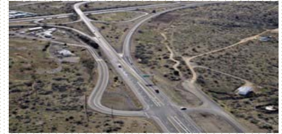
Photo of existing Cordes Junction traffic interchange courtesy of Ames Construction ~ Construction of new TI planned for 2010 ~
